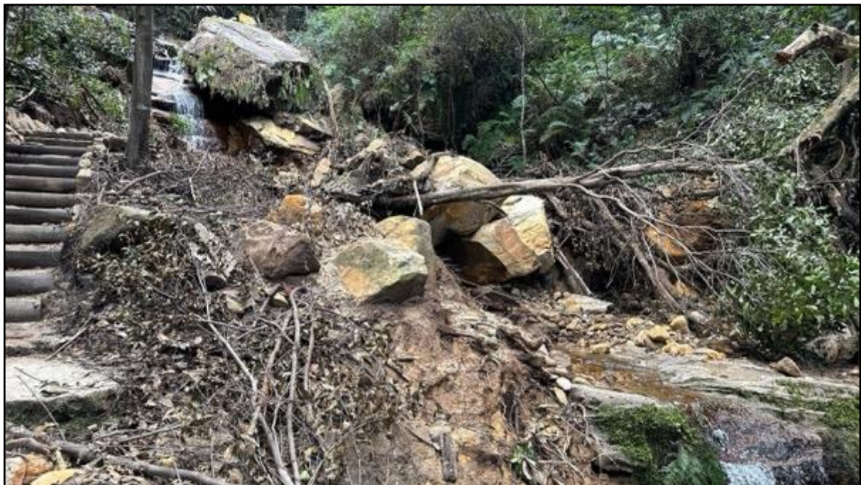
Recent storm damage to Linda Creek.
