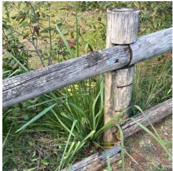
Front fence in poor condition
